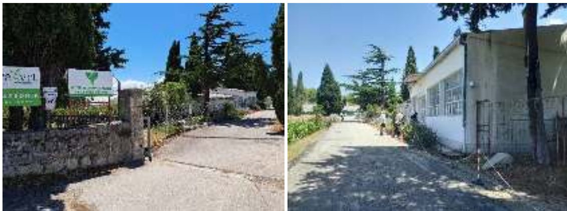
Figure 8. The existing Building A planned for reconstruction
