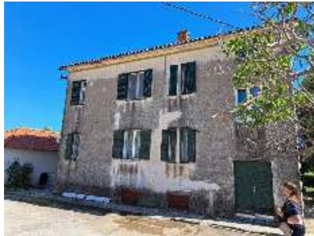
Figure 20. The existing Building 2A planned for improvement of basement and attic
