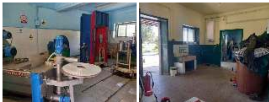
Figure 24. Rooms in the Building 2B
