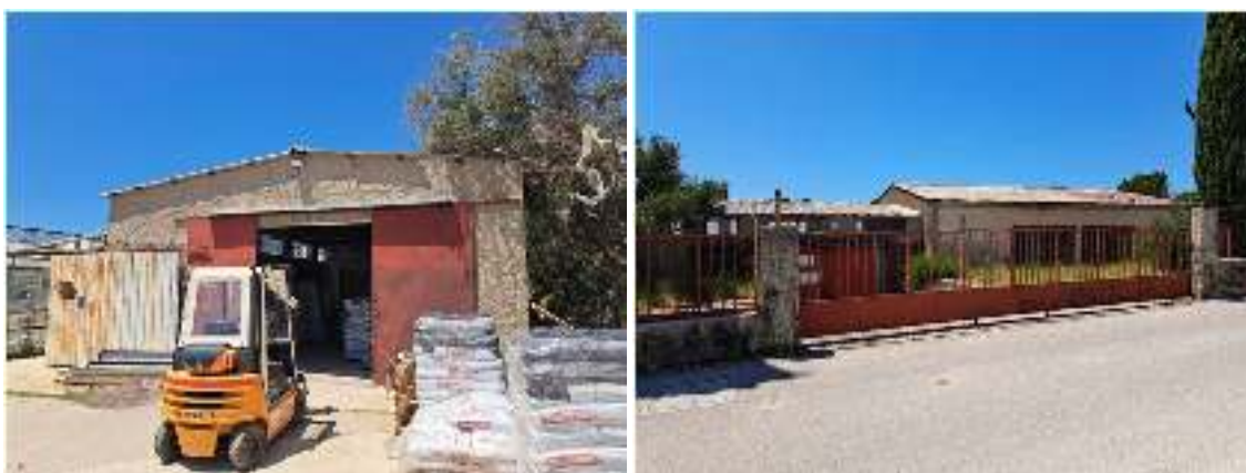
Figure 10. The existing Buildings C and E planned for reconstruction (future Building C)
