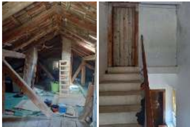
Figure 22. The attic of the Building 2A
